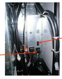
1 - Toggle AC Distribution Box switch to Off position.
